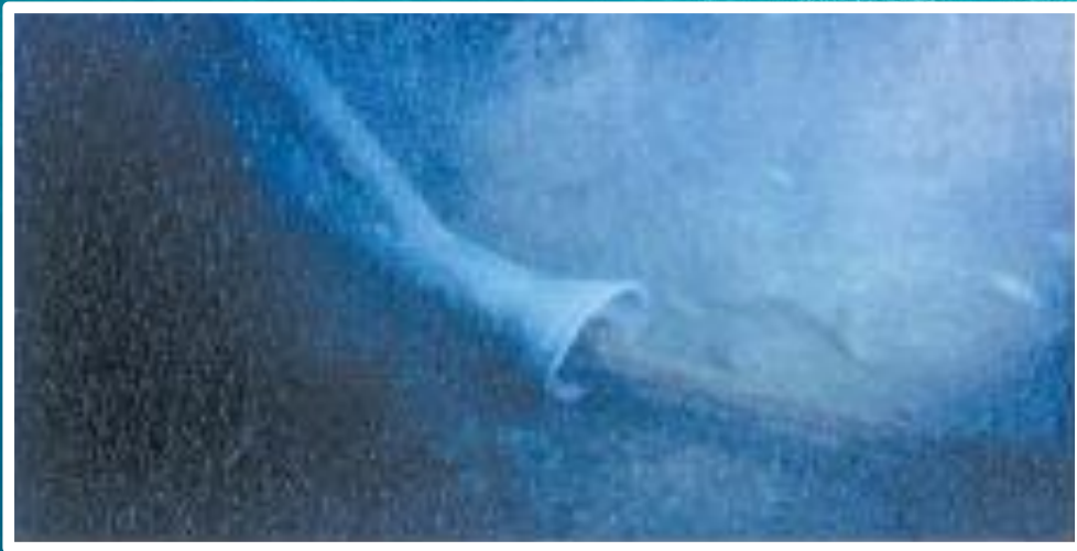
CABLE EXITING J TUBE AT SEABED
