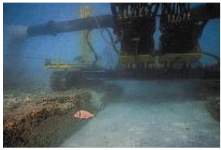
TRENCHER AT WORK
