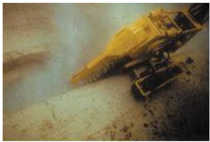
TRENCHER WITH CUTTER AT WORK
